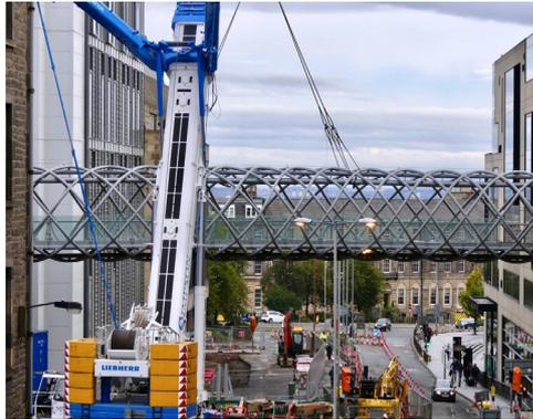
Installed in 2003 as part of the Omni Centre development, the 50m 'complex composite beam' weighed 90 tons and, because its foundations were divided by a geological fault line, was designed to move +/-15mm. If all its circular hollow tubes were straightened out and placed end to end on the road, we estimate they would stretch from their original site nearly to the junction of Inverleith Row and Terrace.
