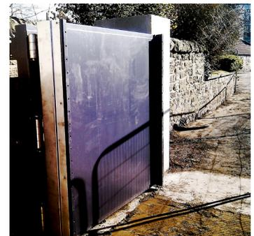
This impressive structure is part of the two giant floodgate sets recently installed on Warriston Road. Reader Neale Gilhooley photographed them, and has been told by the Council that they are required in case water is pushed over the riverside wall due to new, higher defences on the opposite bank.
