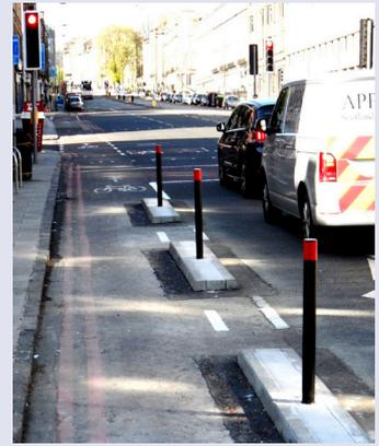
Cycleway delineators, known as 'kerb splitters' (short stretches of kerbs laid back-to-back, with **collapsible/reboundable bollards** in-between) have been installed on Leith Walk at the junctions with **Pilrig and Brunswick Sts.** The previous unfit-for-purpose delineators ('orcans') were removed in a process which **cycling correspondent** Tim Smith terms 'orcastration'.
