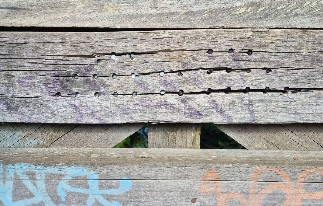
Figure 2: Top chord node – internal view.
