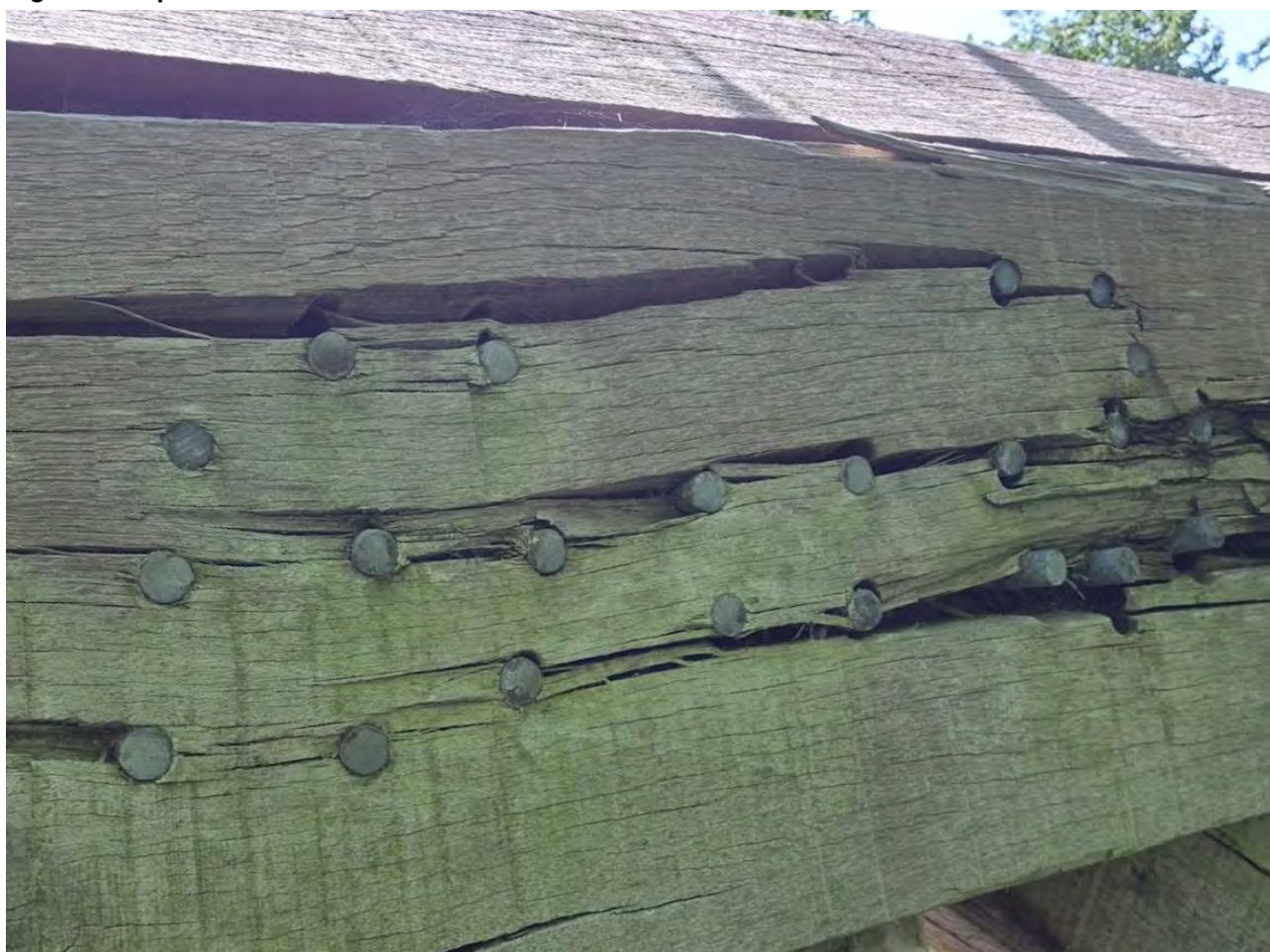
Figure 3: Top chord node – external view
